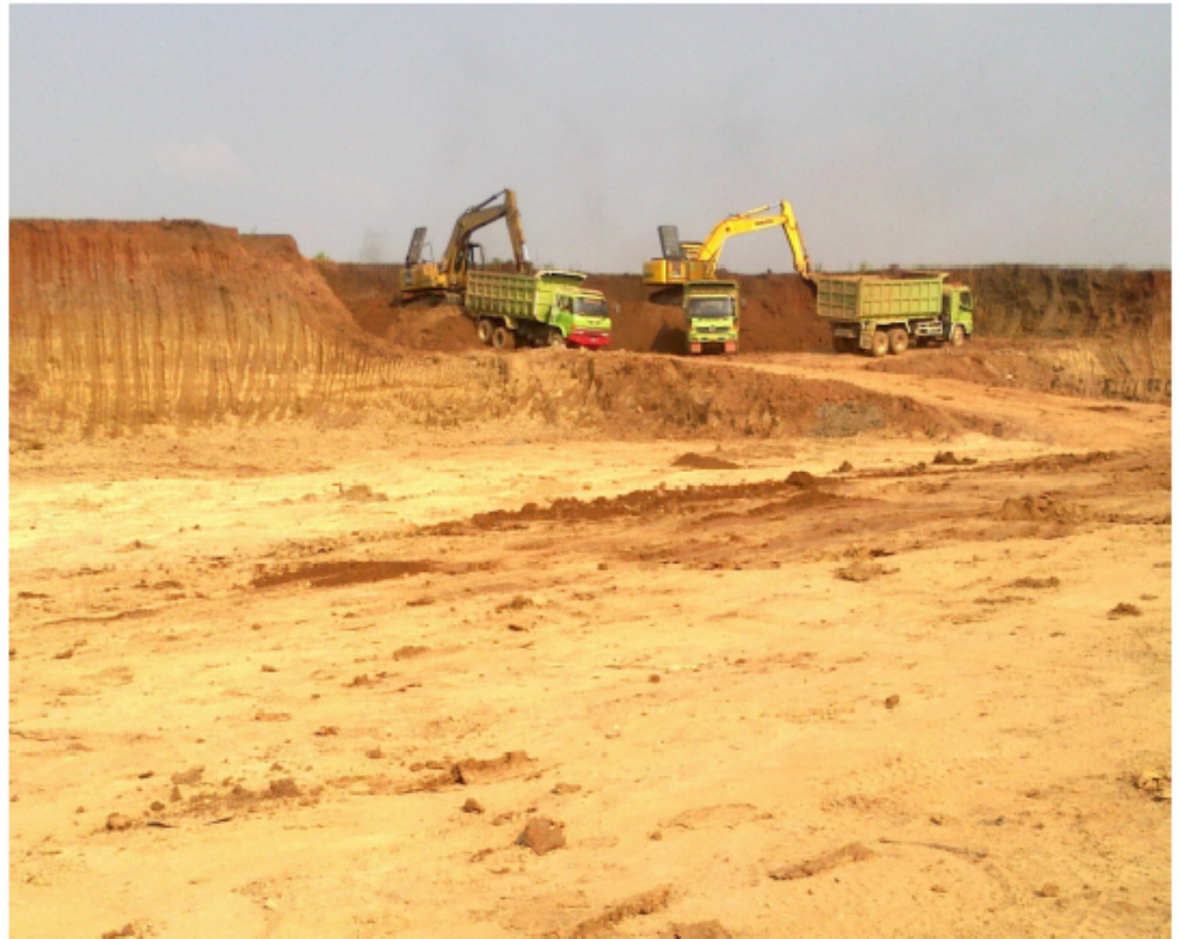
Cut and Fill Work in Phase 3
